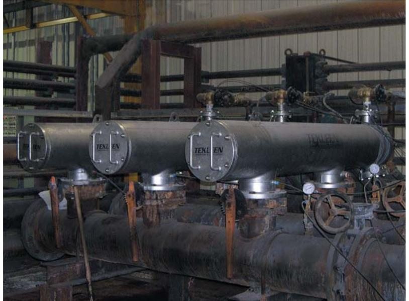
*Cooling Water Filtration at Steel Dynamics, Butler, IN 3,000 gpm,
