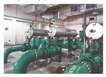
Because they are self-cleaning, and it is an automatic process, there is no labor or downtime required for regular filter cleaning. The filters are made from stainless steel, and consequently there is no risk of deterioration. This means longer equipment life, and no contamination into the water from rust or plastic wear-off.
